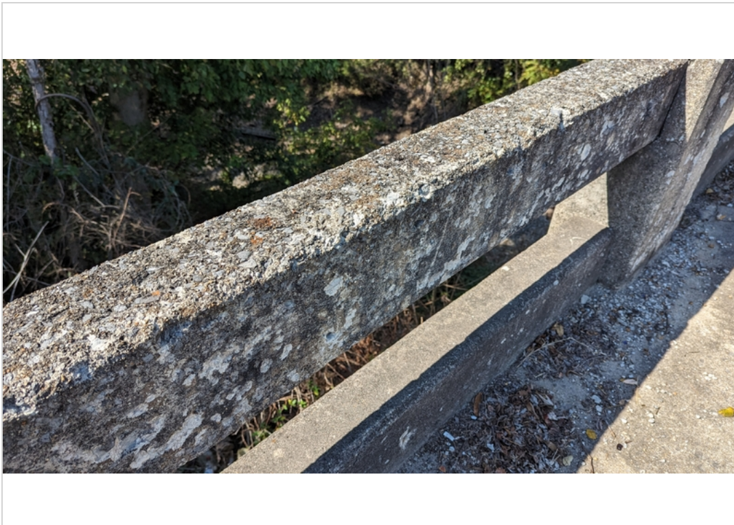
Typical scaling on bridge rail
