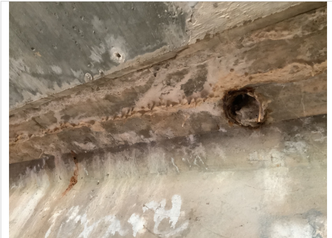
Typical moderate efflorescence in bottom of deck
