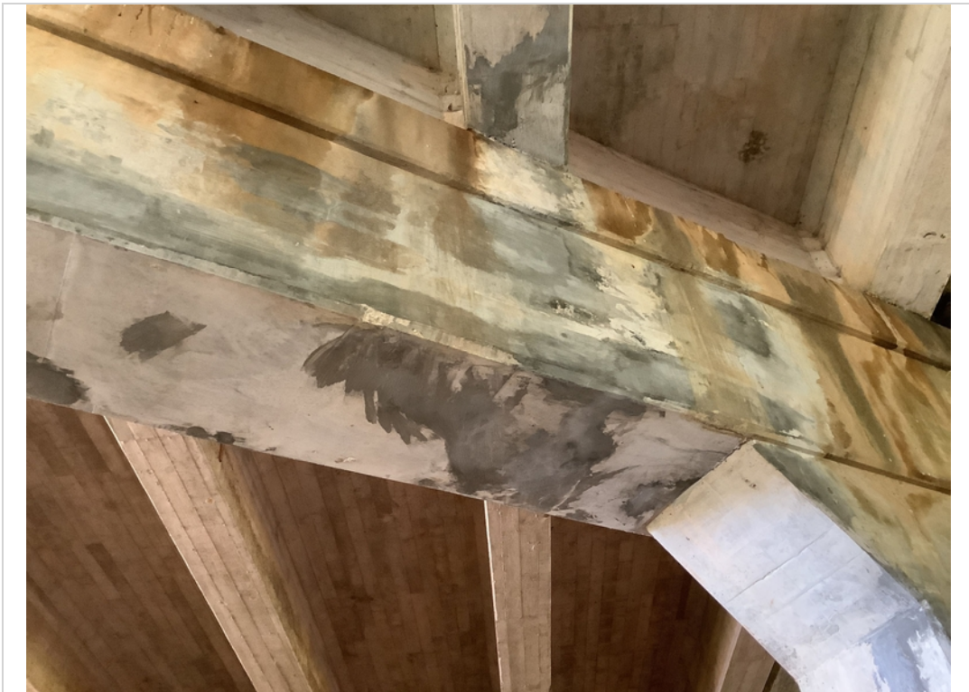
Typical repaired area
