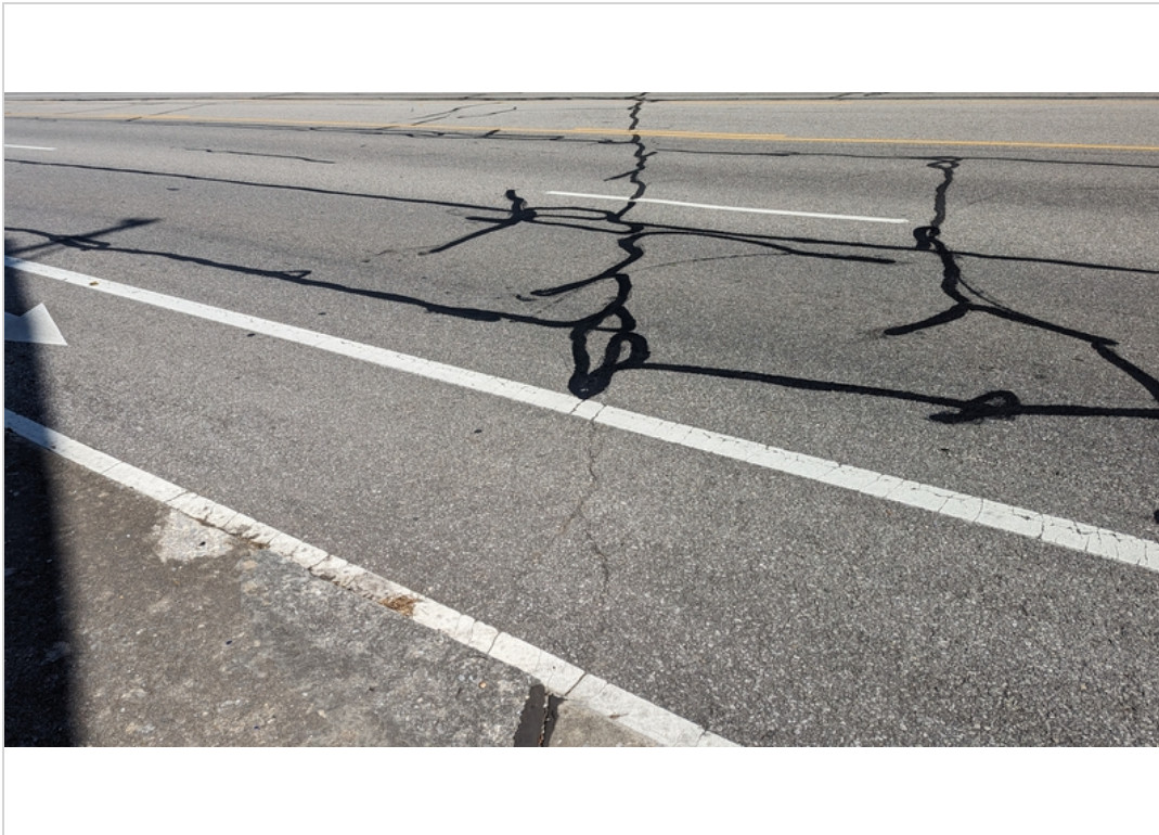
Typical sealed cracks in wearing surface
