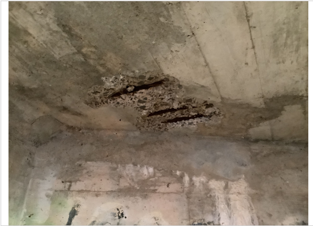
Typical spall with exposed rebar in bottom of deck
