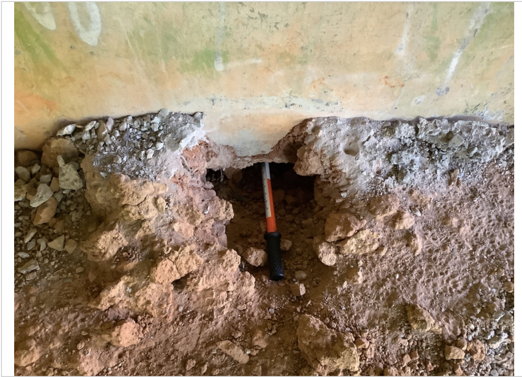
Typical void at abutment #1
