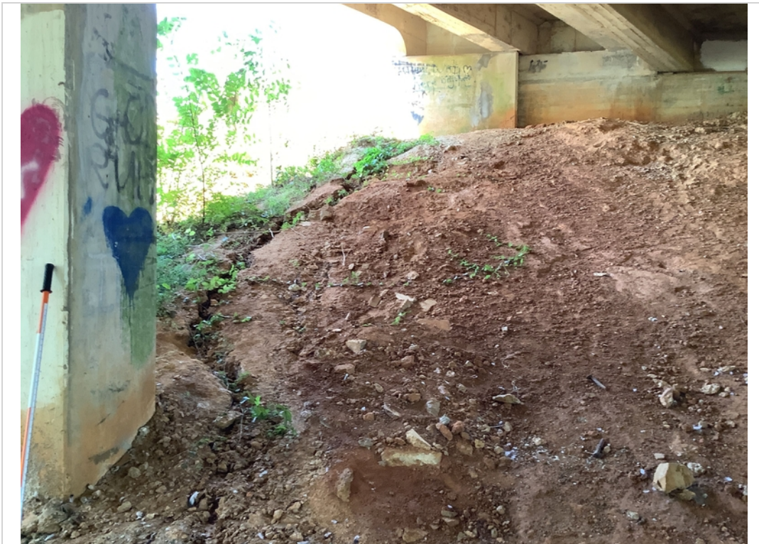
Typical embankment erosion at abutments
