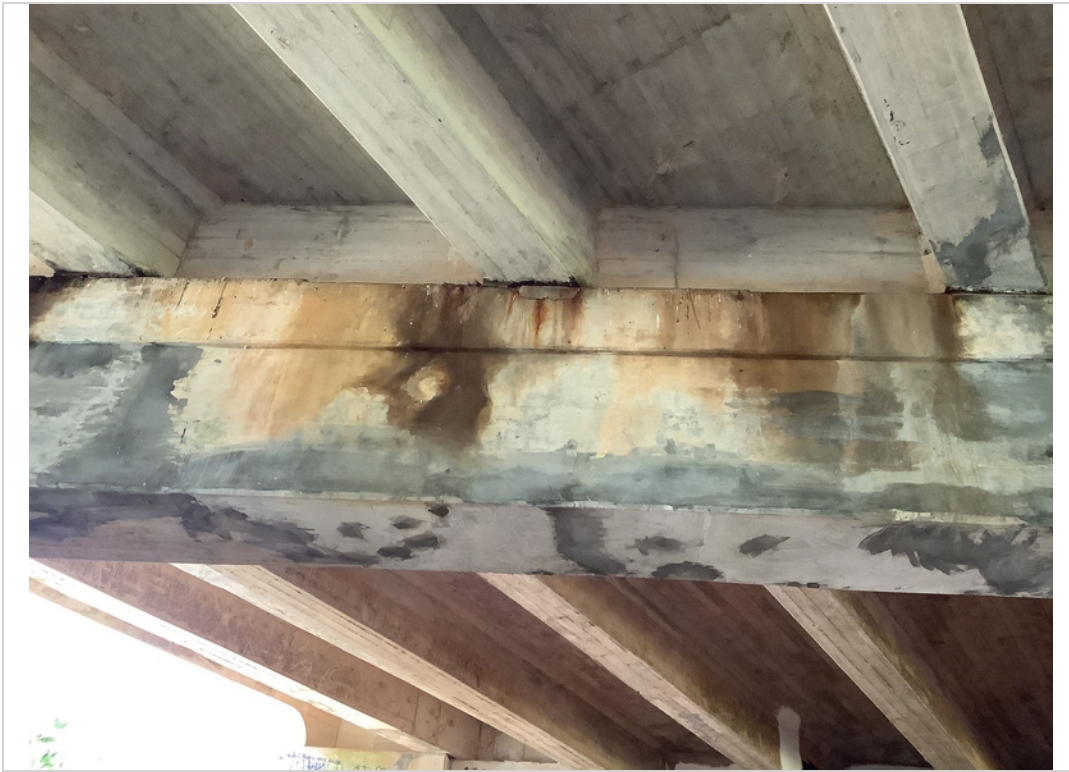
Typical delaminated area
